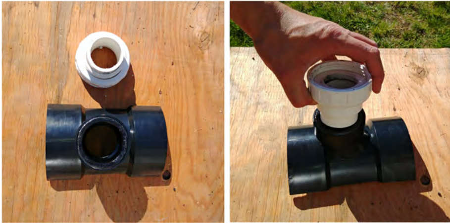
Fig. 33. Installation of the PVC union fittings.
