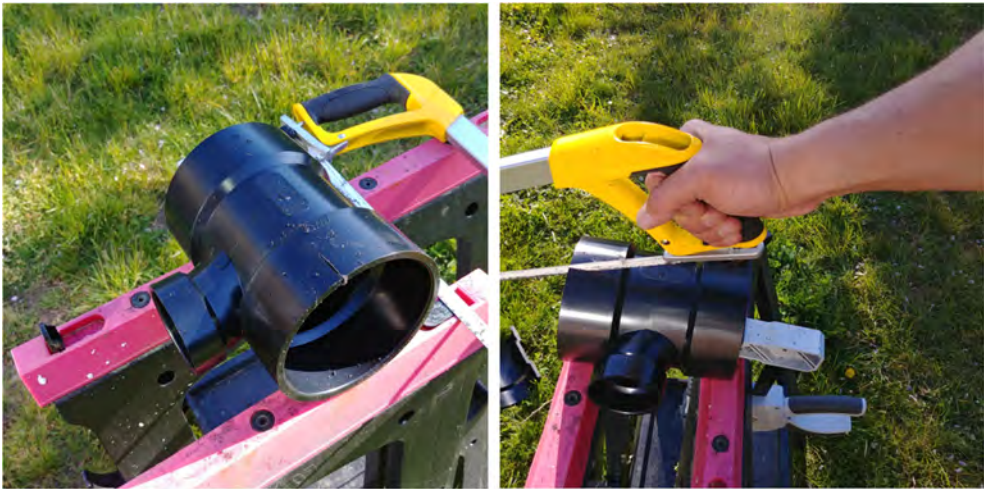
Fig. 31. Cutting of the tee fitting.
